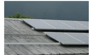
*Panels consistent w/existing slope of roof, on elevation not easily visible from public right of way. credit: Peggy Cox via @wcn247 on Flickr*
